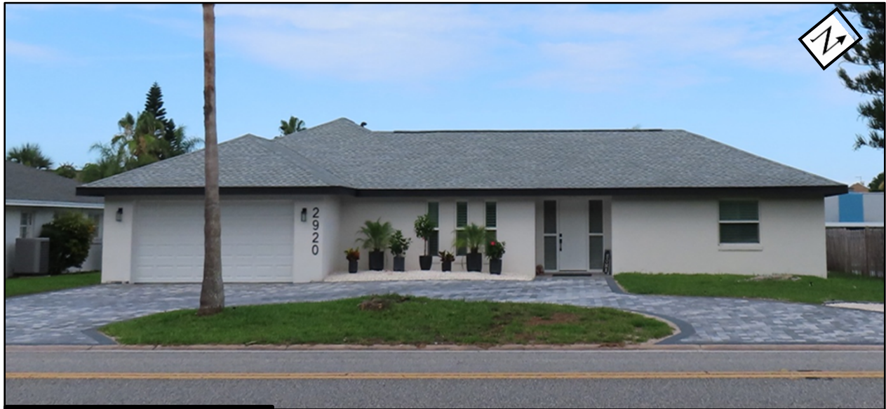
Figure 3: 2920 S. Peninsula Drive Street View
