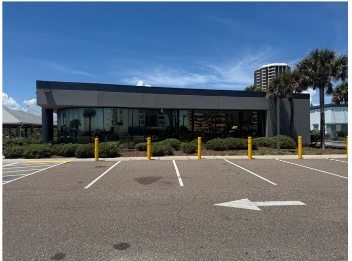
Front of the building
