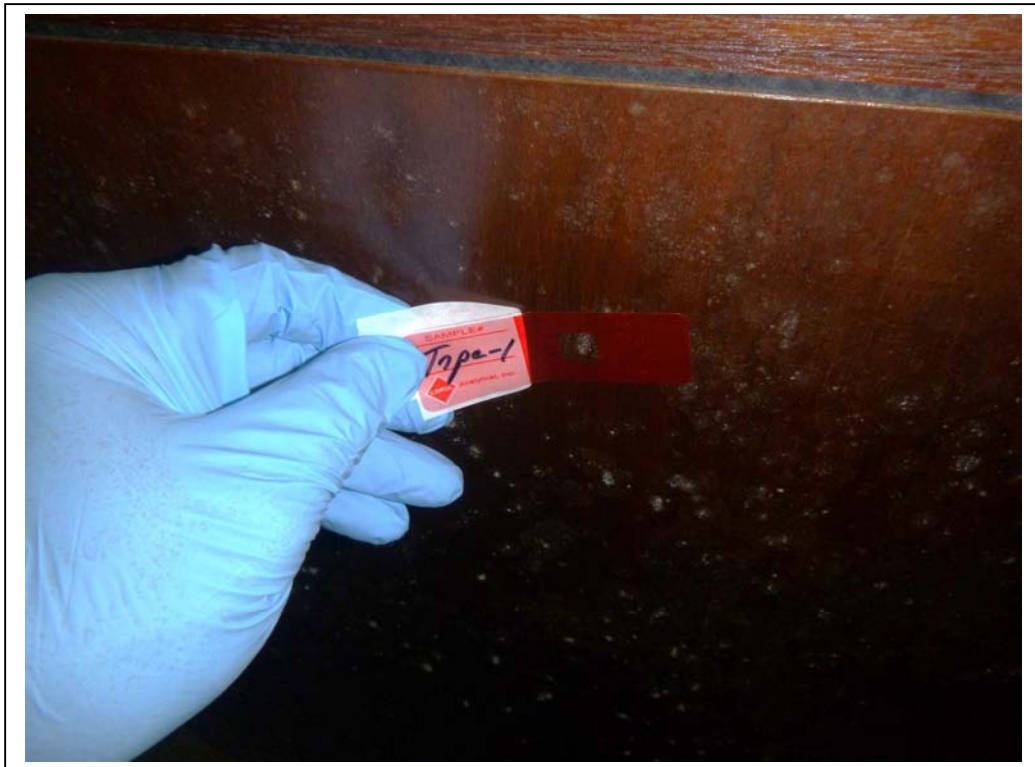
Photo #14; Moldy Desk – Tape Lift Surface Sampling View
