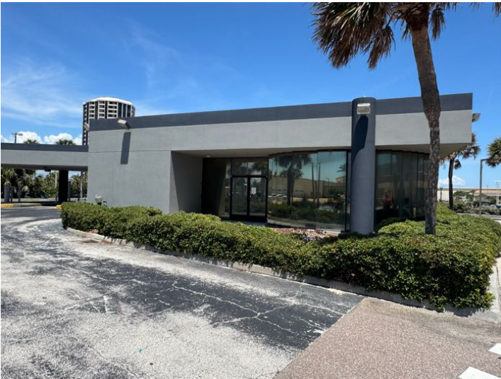
Side of the building
