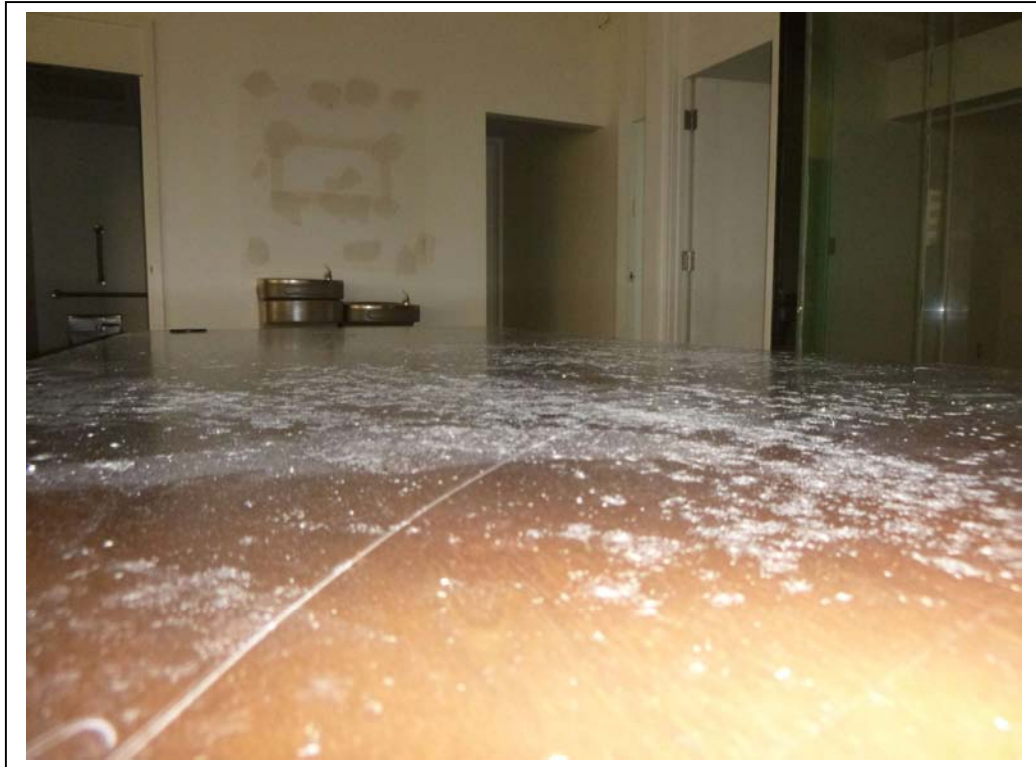
Photo #7; Representative Moldy Desk In Main Lobby View
