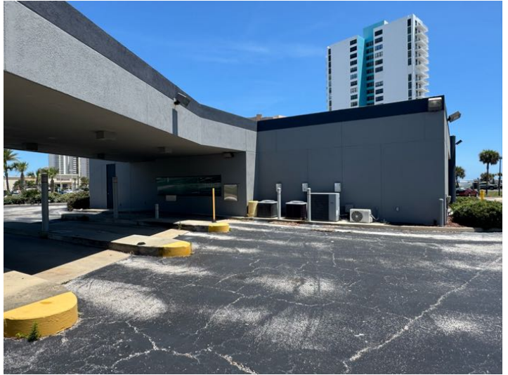
Rear of the building
