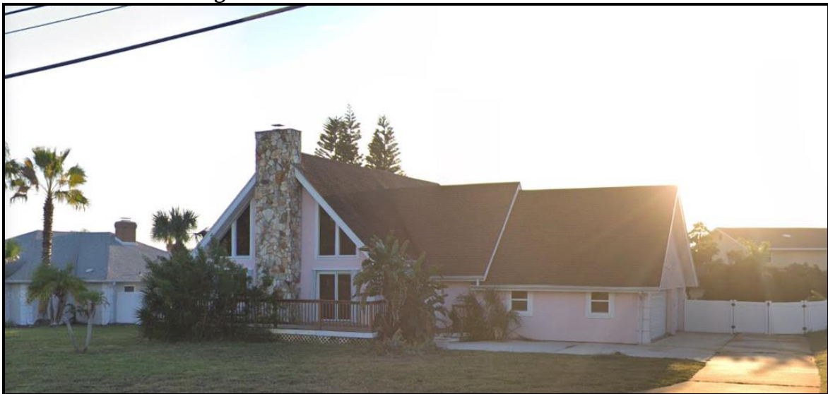
Figure 3: 2924 S. Peninsula Drive – Street View
