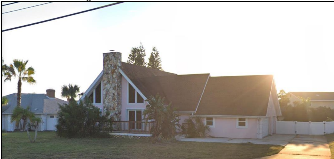
Figure 3: 2924 S. Peninsula Drive – Street View
