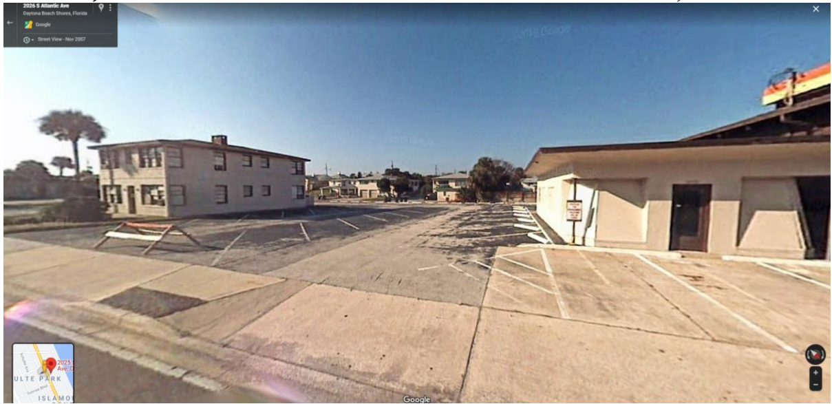
Picture C, 2026-2030 S. Atlantic Ave: TI Maintenance & Westside Rooms; 2007
