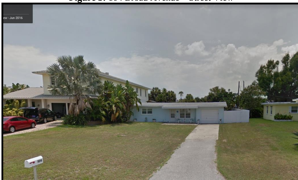
Figure 3: 104 Broad Avenue – Street View
