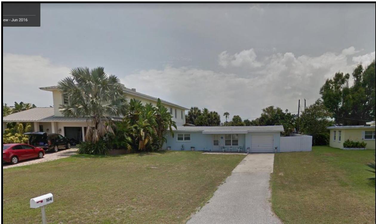
2: Street View: 104 Broad Ave.
