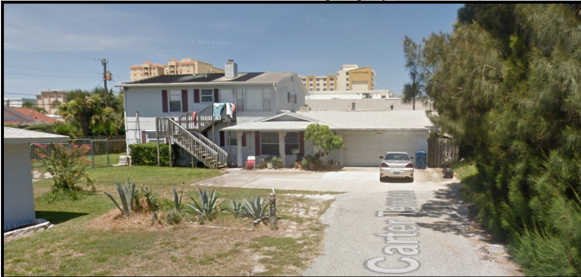
B: Street View of Annexing Property (6 Carter Ter.)
