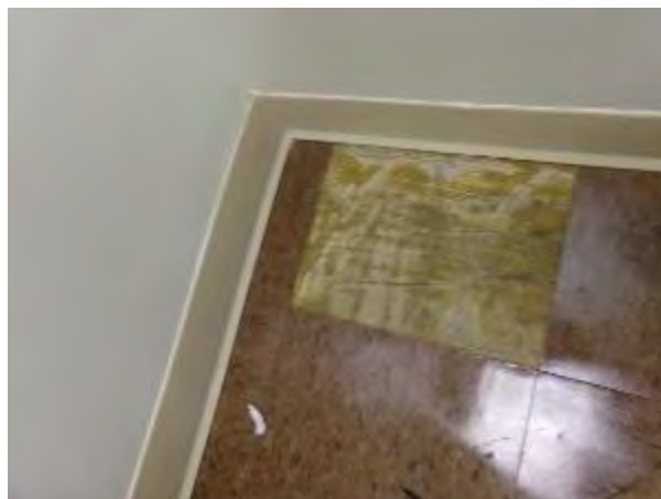
HA-24: Brown 12' x 12' Vinyl Floor Tile; HA-25: Yellow Floor Tile Adhesive
