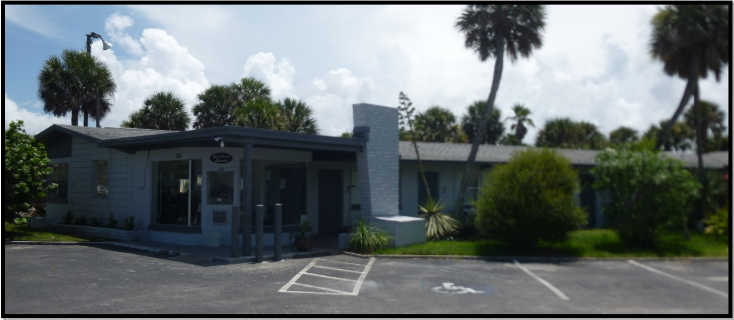
View from northeast of property
