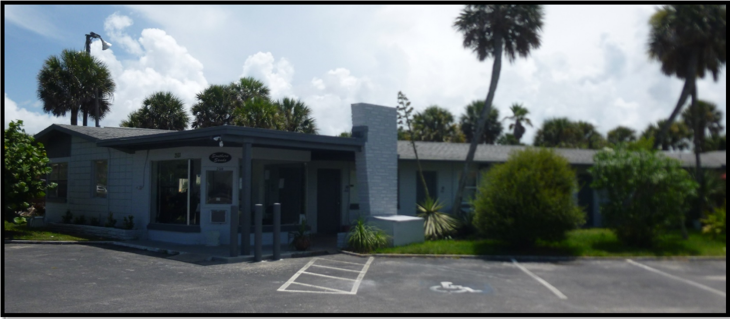
View from northeast of property
