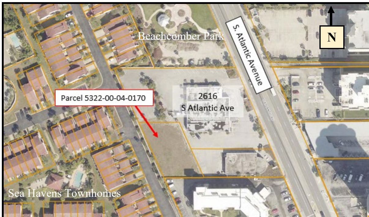
Figure 2: Aerial View of Parcel 5322-00-04-0170 and Surrounding Development
