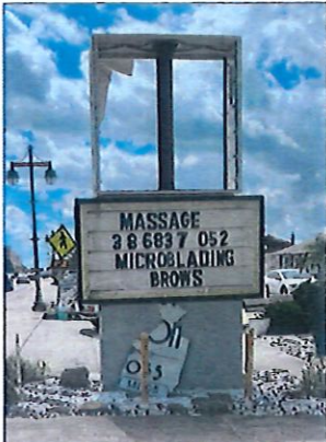
Existing pylon sign to be removed & discarded Pipe to be cut @ grade
