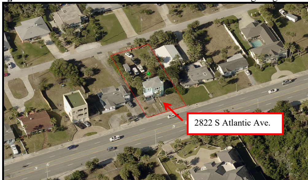
Figure 1: Aerial View-2822 S. Atlantic Avenue and Surrounding Neighborhood
