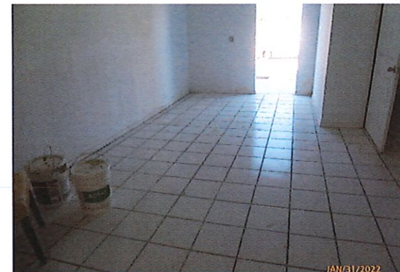
Re- Inspection January 31, 2022
