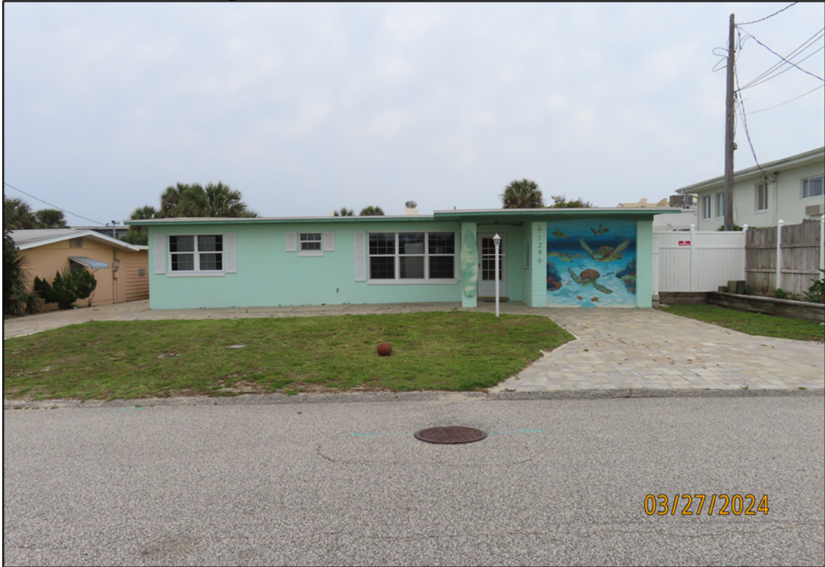
Figure 3: Street View: 129 Esmeralda Avenue
