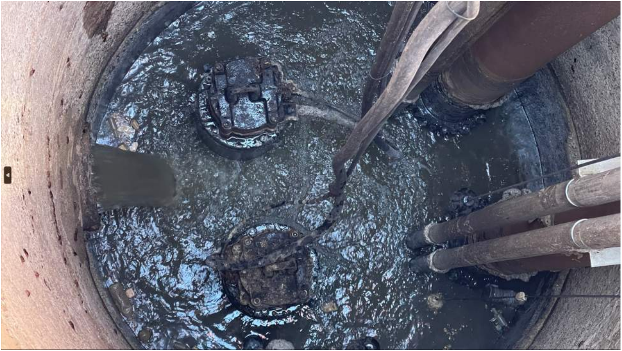
Figure 4-15 Lift Station 5 Unlined Wet Well
