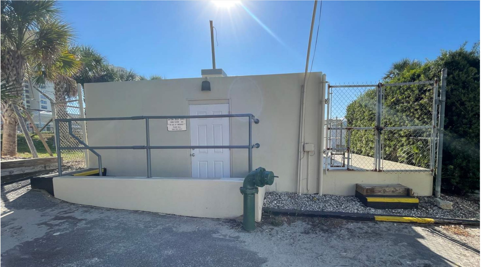
Figure 4-11 Lift Station 4 Building with Narrow Entrance
