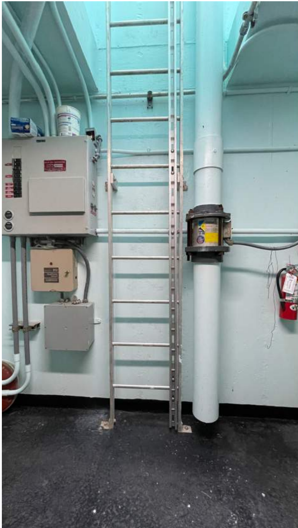
Figure 4-5 Lift Station 1 Dry Well Access Ladder
